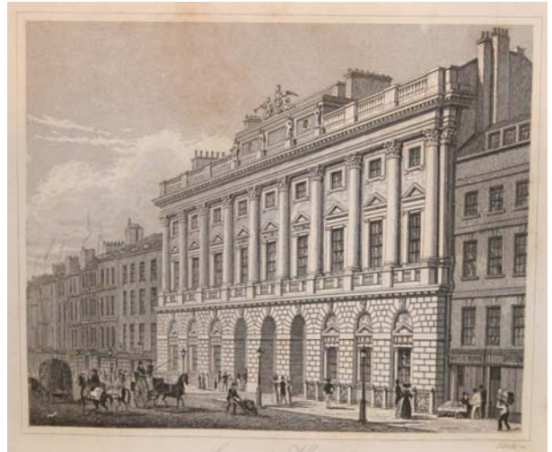
Engraving by Robert Sands in: The Public Buildings of Westminster Described C.I. Johnstone London: John Harris, 1831 [Martin Coll.] 007
